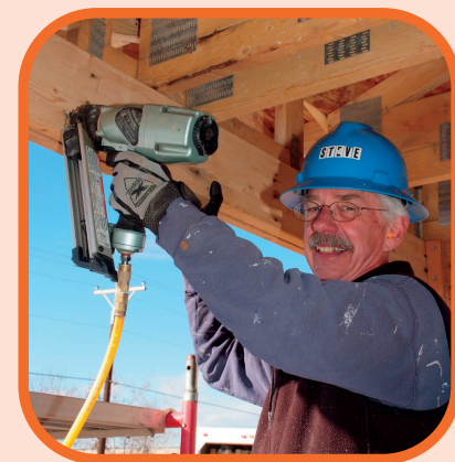
Steve on a Habitat build
